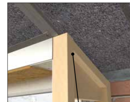
Infill 95 x 362mm In this case infill option is shown as timber. Intrusion panel is cut to accommodate the infill.
